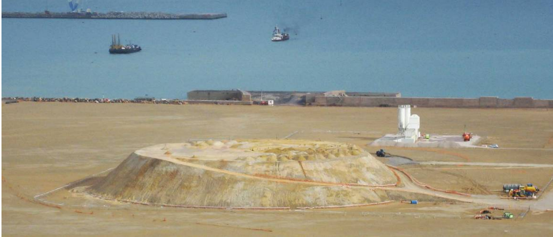
Photo 2: Completed Preload of Tank Nr 1
